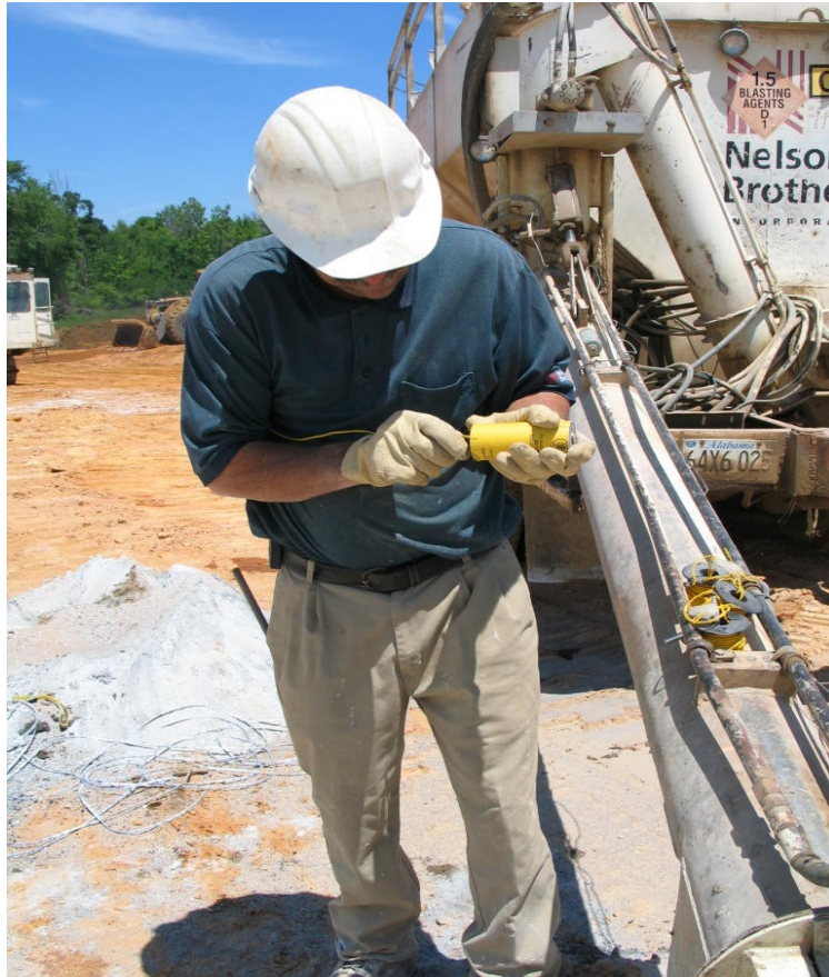
Figure 5 - Preparation of Primer for Blast Hole Loading
