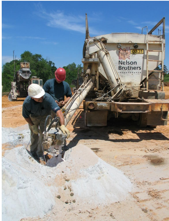
Figure 6 - Loading a Blast Hole with ANFO
